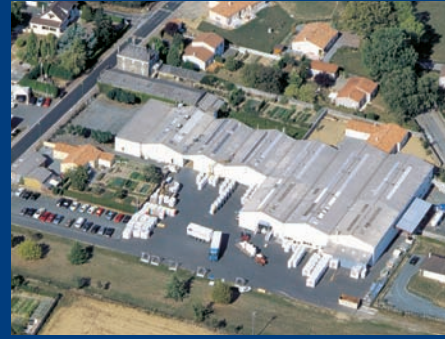
Assembling and dispatching
